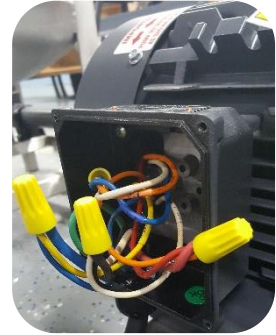
Pump wiring example using wire nuts to form jumpers
